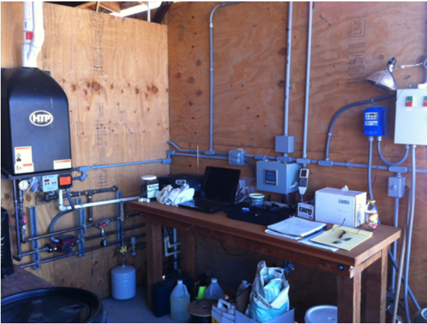
Figure 3-6. The digester control center.
